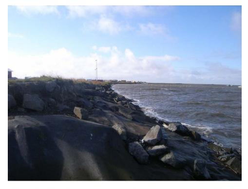
N 59° 56.308' W 164° 02.572' Kipnuk RIMG0132 Photo 1: Looking downstream at the riprap. This project has failed with most of the protection being provided by the fabric at this point.
