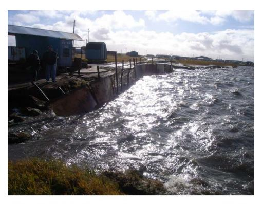
N 59° 56.499' W 164° 02.478' Kipnuk RIMG0095 Photo 1: Looking downstream from sheet metal barrier north of town. Sheet metal barrier is attached to a 2 inch pipe driven into the ground.
